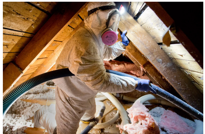
Photo of attic insulation from Efficiency Maine
