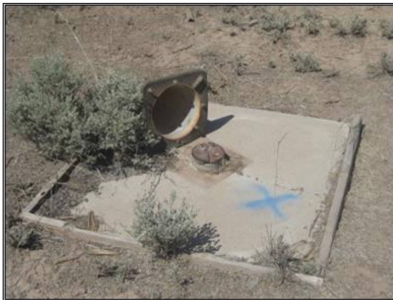
Figure 44: Example of an Improperly Abandoned Well (CRWA)
