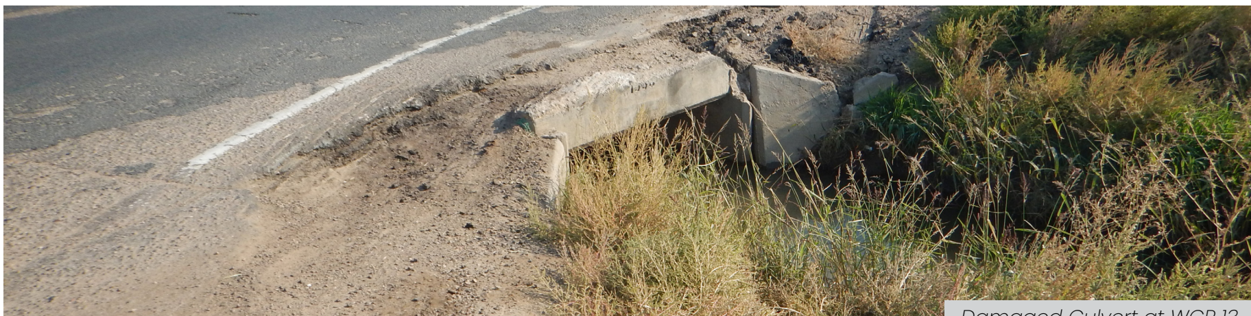
Damaged Culvert at WCR 13
