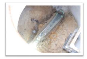
The photos show the presence of grease in the line. Grease is not a permitted discharge, and can cause serious issues (and expensive repair or reconstruction) throughout the sewer system.
