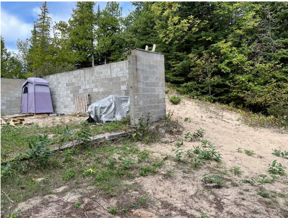
Northern foundation established foundation wall.
