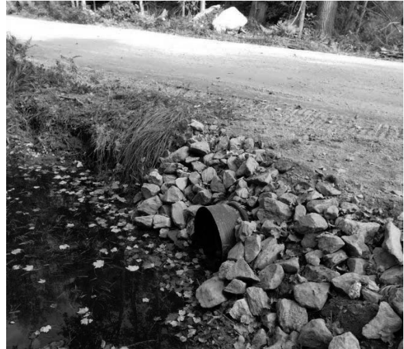
Newly Installed Culvert
