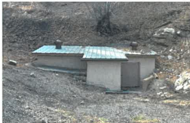
Griffith Spring House.
