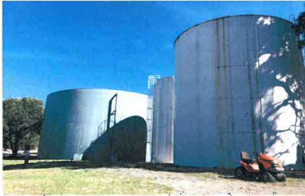
Spring Reservoir, Spring Tank #2 and Spring Tank #1.
