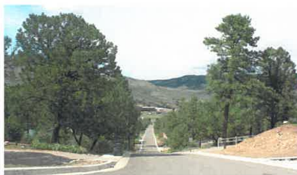
New pavement, curb, and gutter on Dipaolo Hill Drive.
