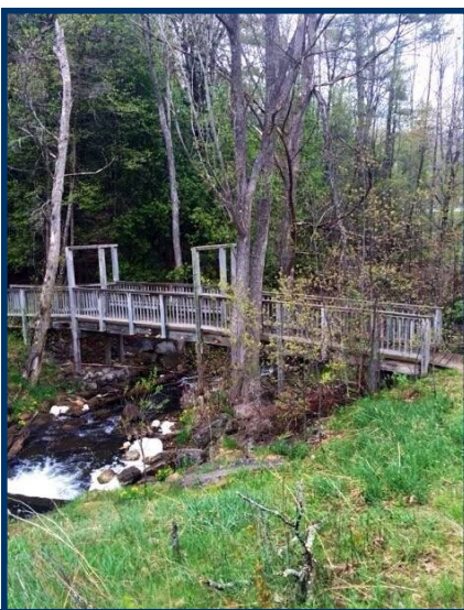
Mayfield Pond Park in Paradise Township.
