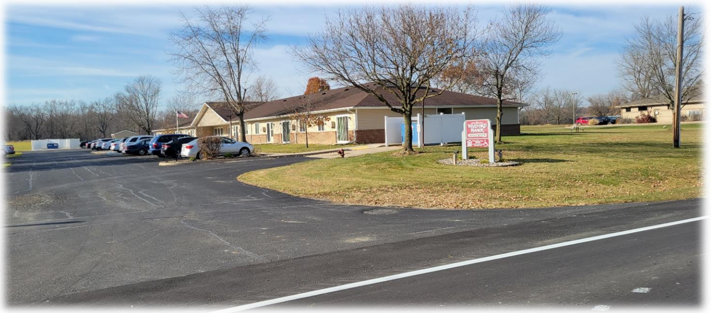
Wexford Manor Apartments
