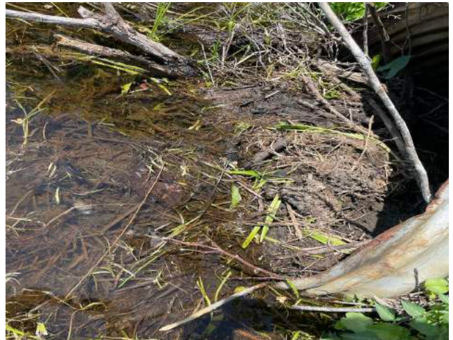
Photo 2 (6/15/22) View of debris plugging the upstream side of Fresh Pond's outlet culvert.
