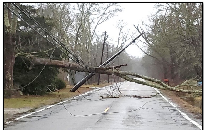
Figure 7-1 Tree Collapses on Power Lines (February 2022)
