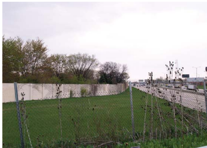
Location of former I-294 ramp
