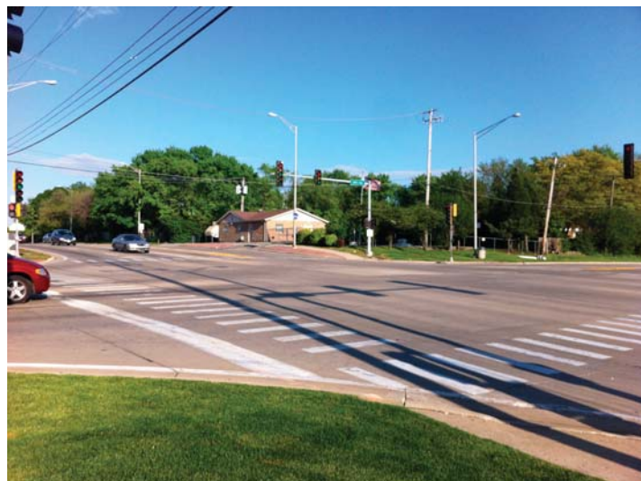
Recent streetscape/intersection improvements in the Village.
