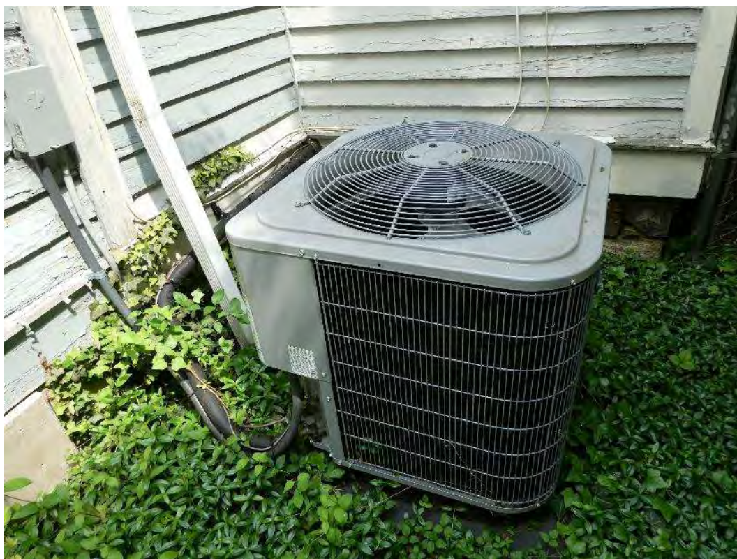
Photograph 23: Exterior condensing unit
