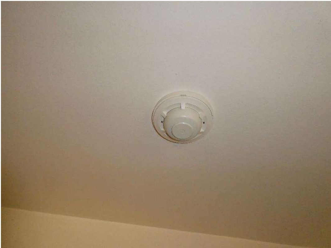
Photograph 31: Smoke detector
