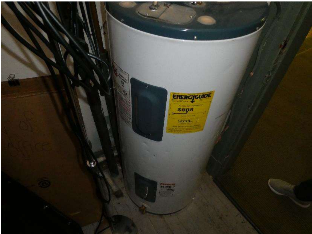
Photograph 29: Electric domestic water heater
