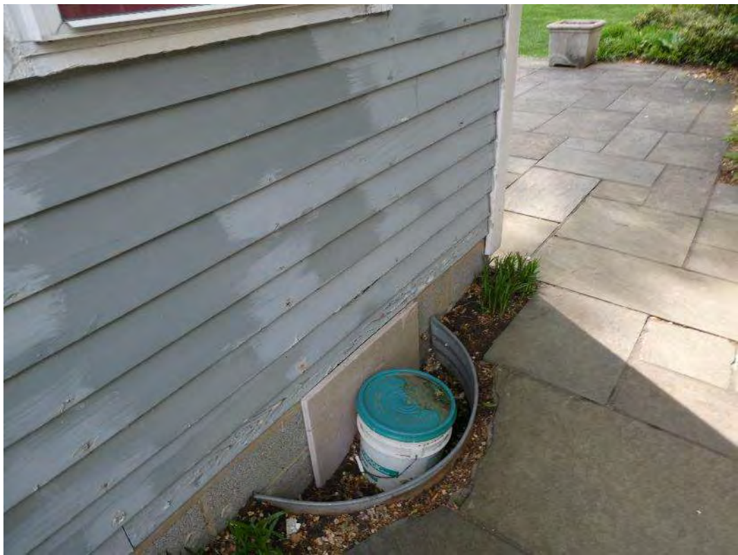
Photograph 10: Blocked sub-floor ventilation
