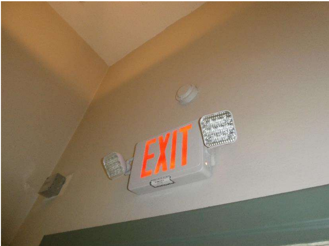
Photograph 30: Fire exit signage and egress lighting
