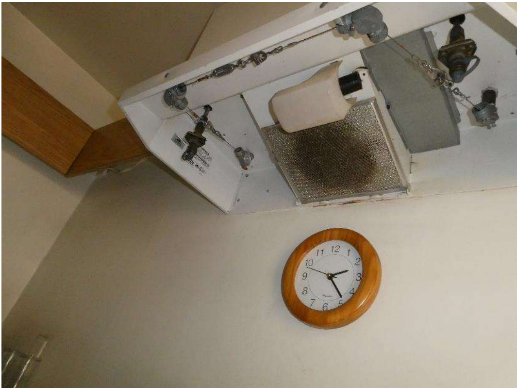
Photograph 32: Chemical suppression system above range hood
