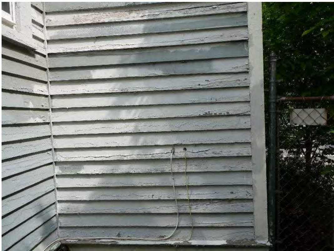
Photograph 14: Deteriorated wood siding
