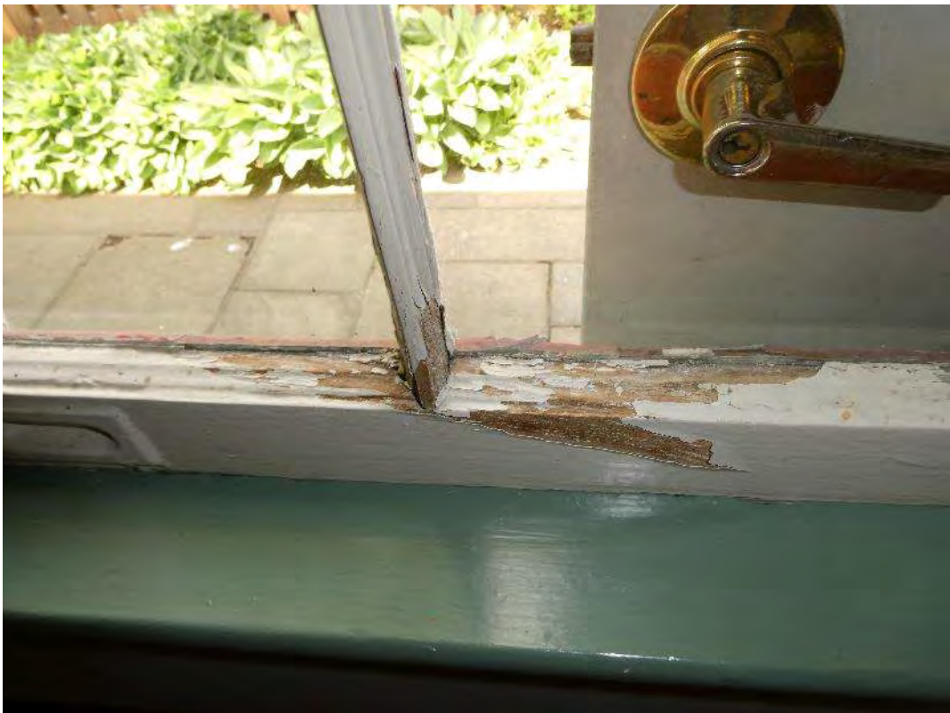
Photograph 15: Damaged windows, viewed from interior areas
