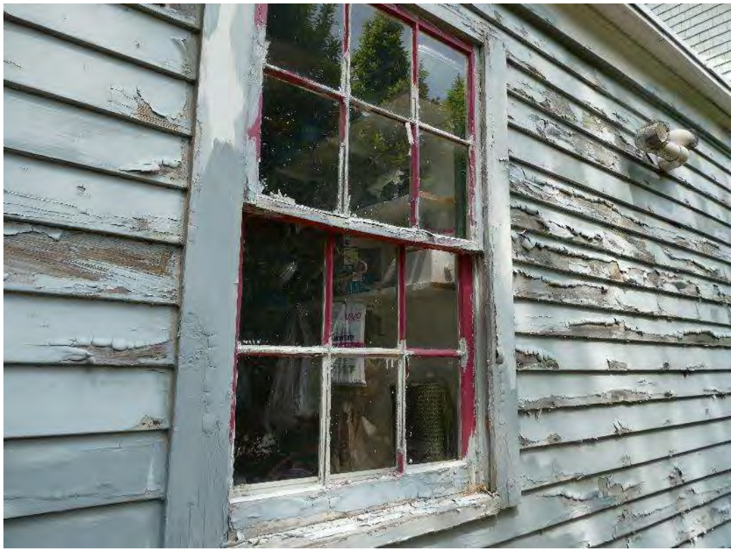
Photograph 13: Deteriorated paint and wood finishes to exterior
