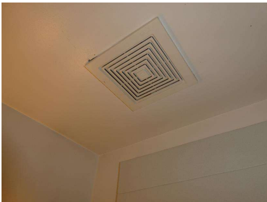
Photograph 24: Exhaust fan in restroom
