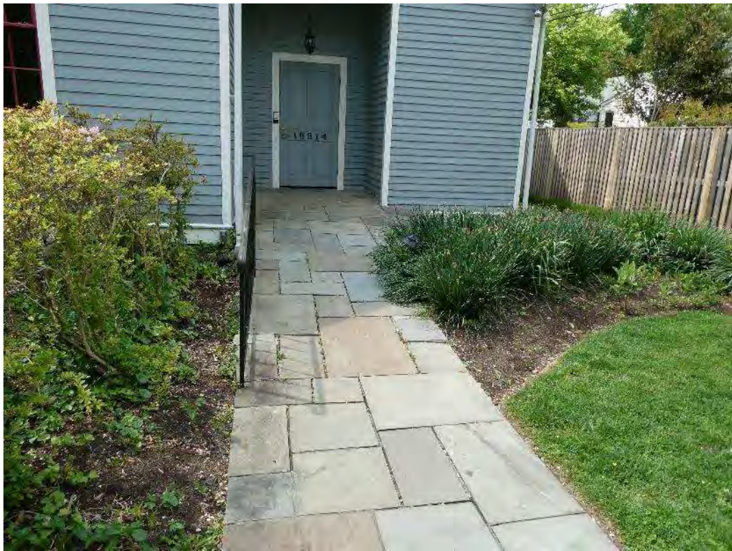
Photograph 1: Ramp at entrance which is not ADA compliant
