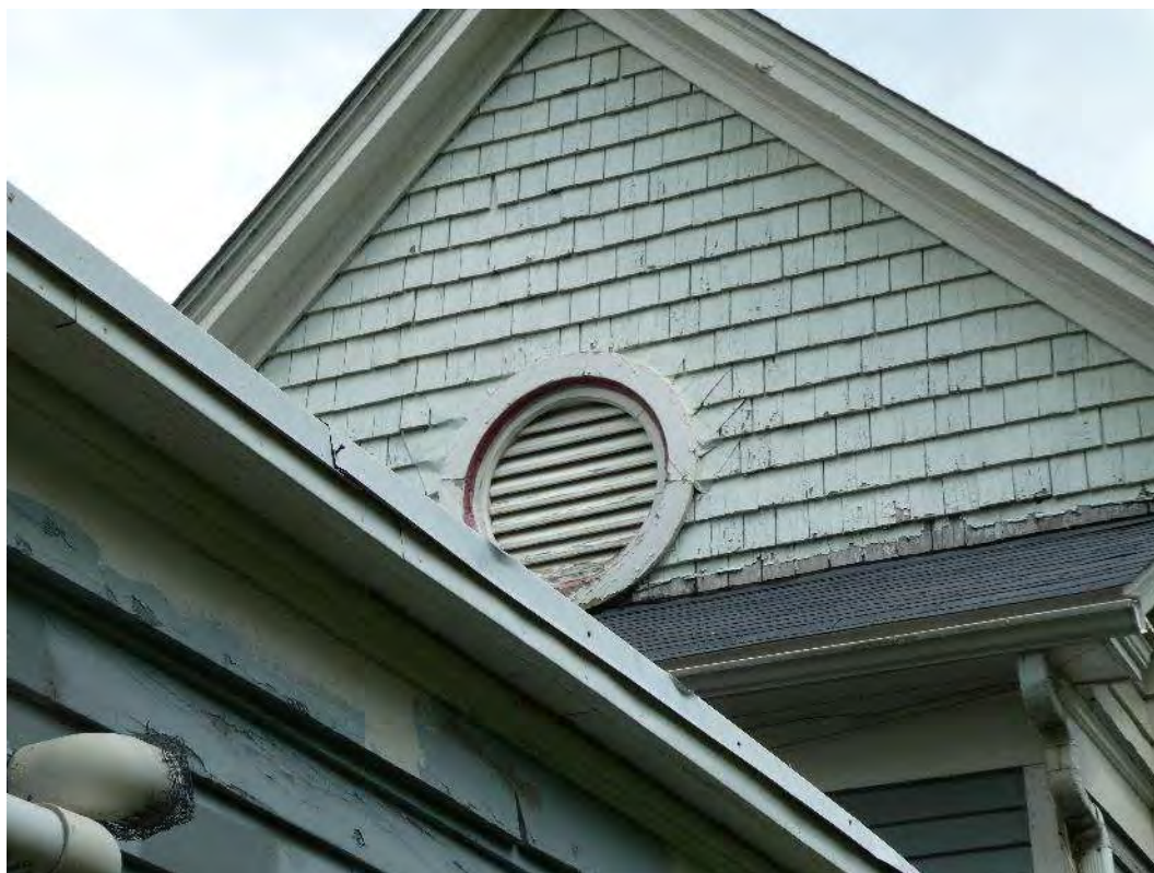
Photograph 17: Deteriorated wood shingles to wall at apex
