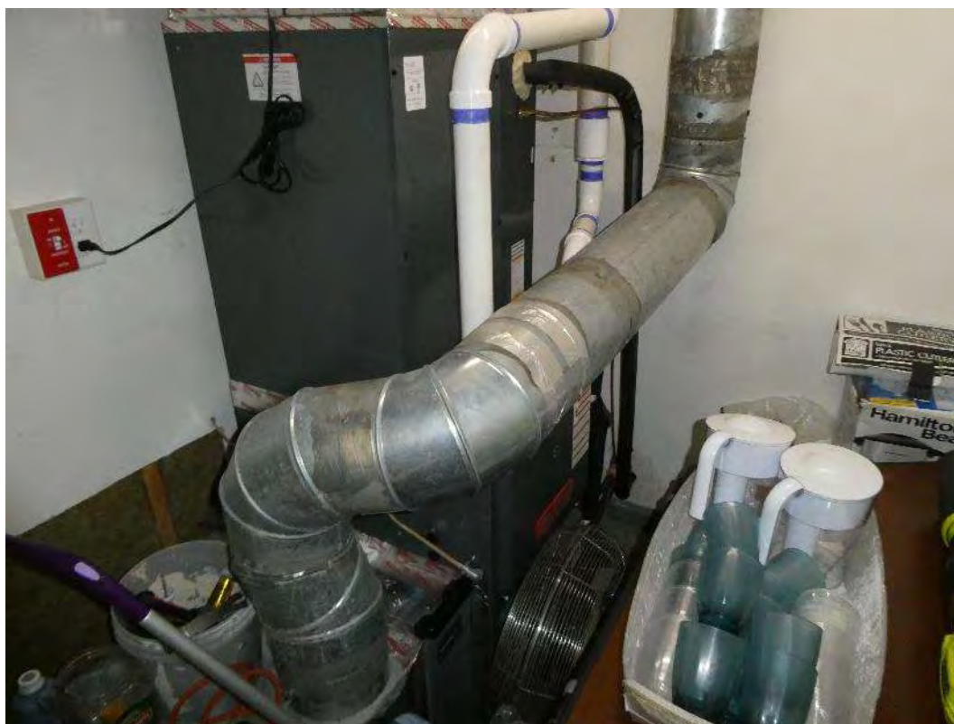
Photograph 21: Gas furnace in closet area serving rear of building
