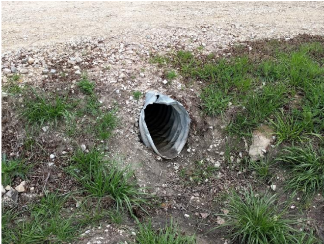
Figure 7C: Culvert with minor damage
