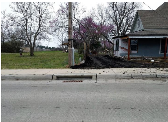
Figure 7B: Curb and Area Inlet
