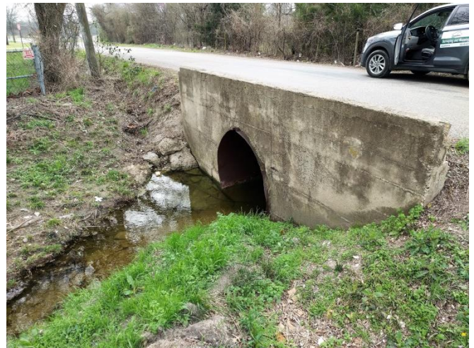
Figure 7D: Culvert with headwall
