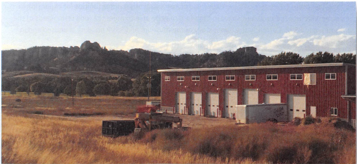
Crawford's new fire hall nearing completion in September 2017
