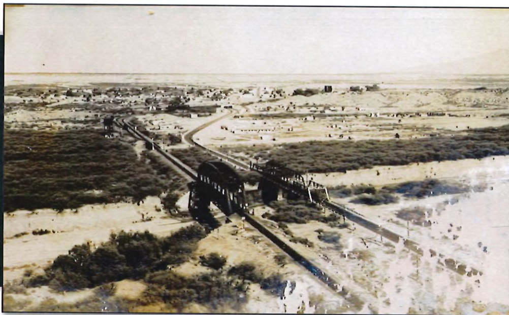
Figure 1. View of the San Pedro Bridge in Benson, no date (Benson Historical Museum)
