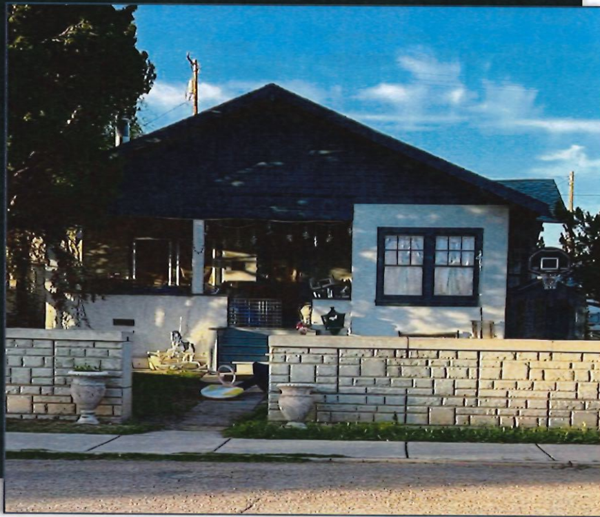
Photograph 4. View of 193 West 6th Street showing the Craftsman Bungalow architectural style found in the Apache Powder Historic District (Cindy Allen)
