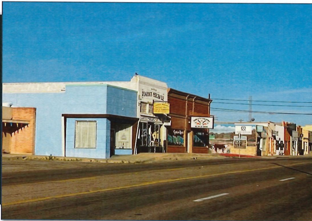
Photograph 1. Current view of 4 th Street, looking southwest (Cindy Allen)
