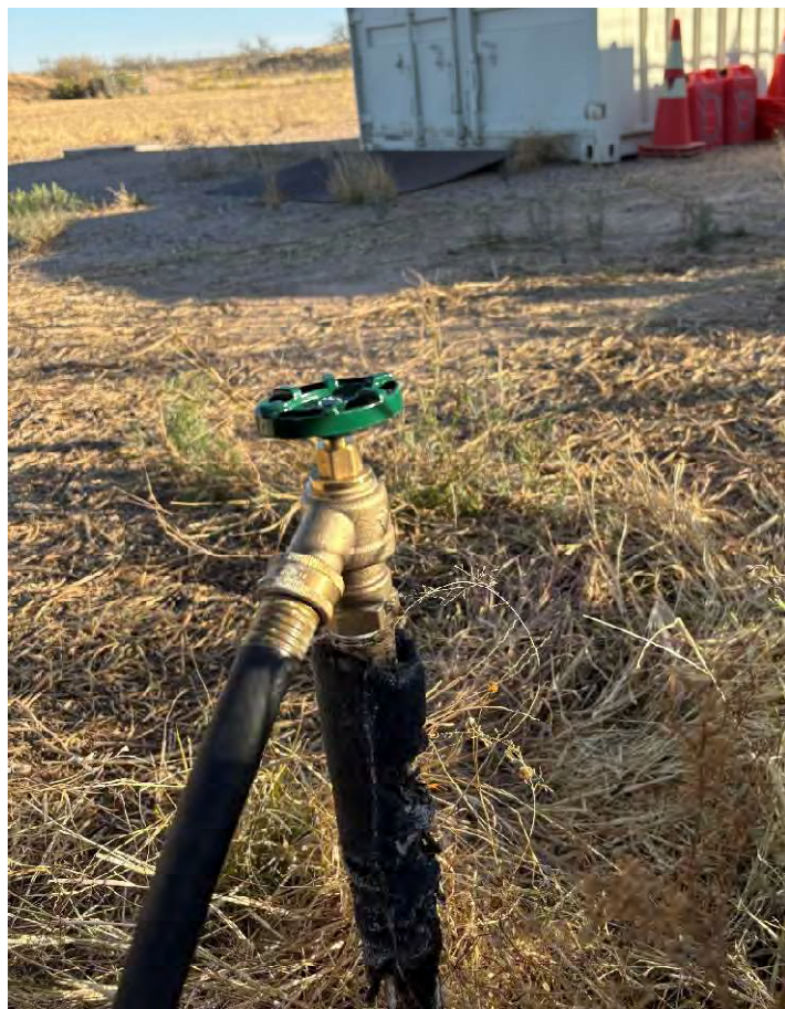
Figure 2 - Water valve after repair
