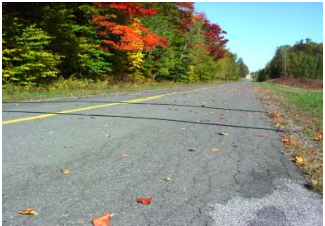
Traffic Counts Burgess Road, Hayes Township
