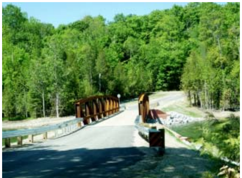
The New Holy Island Bridge , June 2009
