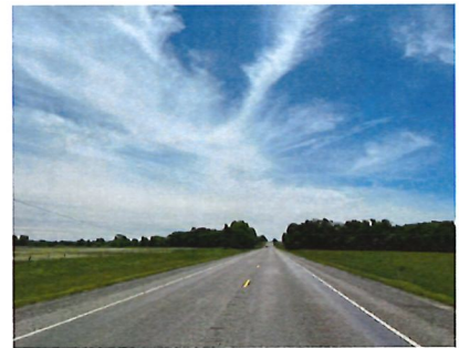
Most of the roadways in Canton have a rural character, with open drainage and no pedestrian facilities.
