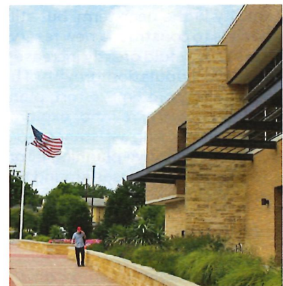
Community centers provide places for social gathering and community building.
