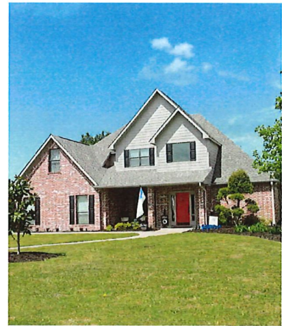
Existing single family homes in Canton range in size and scale.
