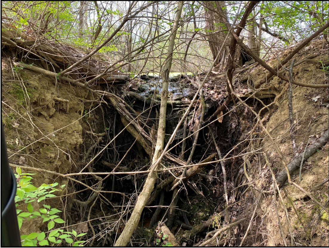
Photo 9 – Westerly view of a spillway observed within the earthen berm along the eastern boundary of Wetland 1. This spillway provides a surface water connection from Wetland 1 to Stream 3.
