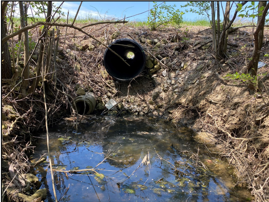
Photo 36 – Westerly (upstream) view towards the beginning of Stream 1. Stream 1 originates at the outfall of a round corrugated plastic culvert beneath N. Old State Road.
